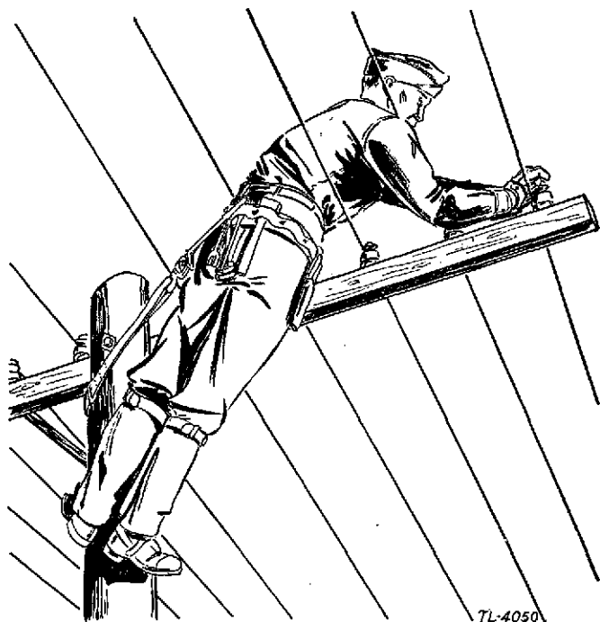
FIGURE 75.—Working on outer wire of cross arm.
